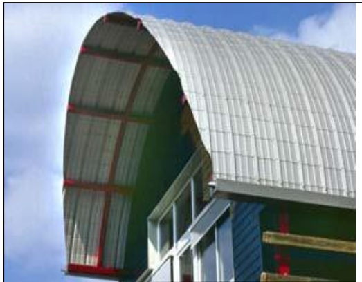
Curved roof with galvanized steel sheet
