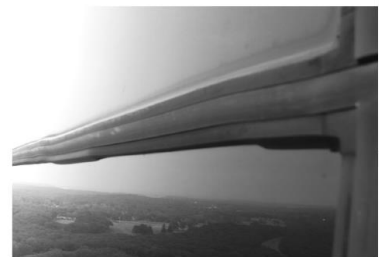
Figure 20: Gaskets disengaged from glazing
