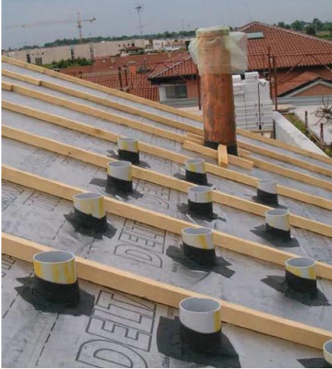
Sealing of curved elements (aerators) by elastic adhesive strip.
