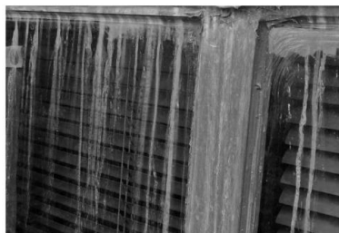
Figure 19: Streaked glazing
