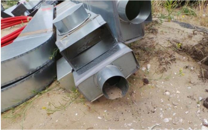
Unprotected storage of ducts
