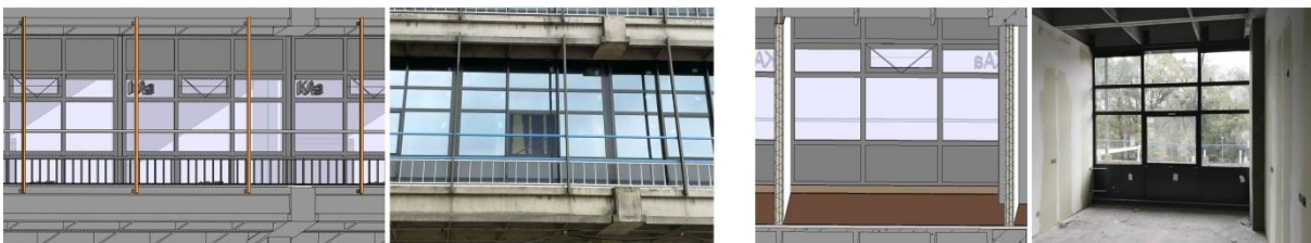
Figure 7: Comparisons between real live situation and the BIM model: general outside and inside views on the façade panels
