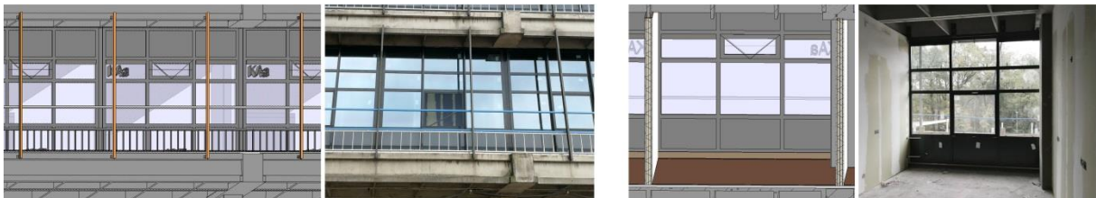
Figure 37: Comparisons between real live situation and the BIM model: general outside and inside views on the façade panels
