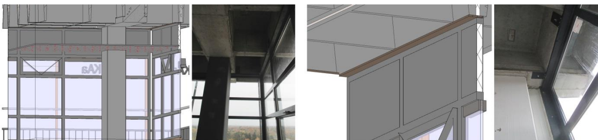
Figure 38: Comparisons between real live situation and the BIM model: corners in a corner room and middle room
