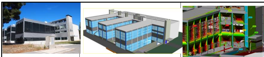
Figure 4: Different views of Cartif III building
