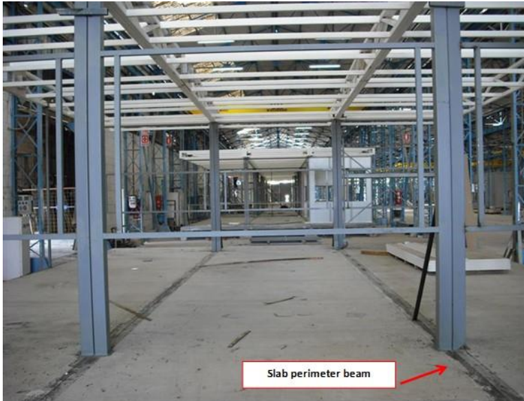
Figure 68: slab perimeter beam
