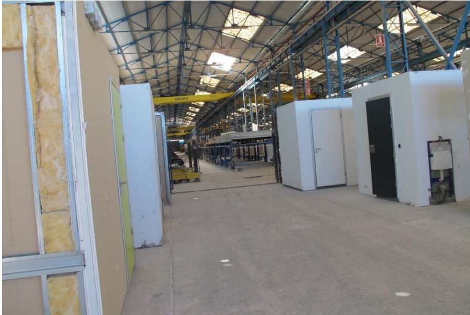
Figure 58: Industrial buildings for manufacturing and storage
