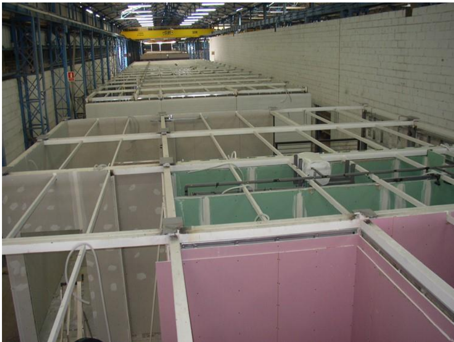
Figure 63: Industrial buildings for manufacturing and storage
