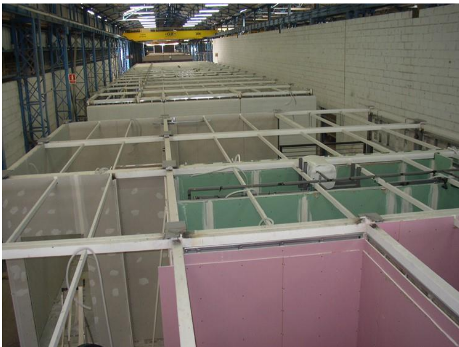
Figure 65: Modules assembly off-site
