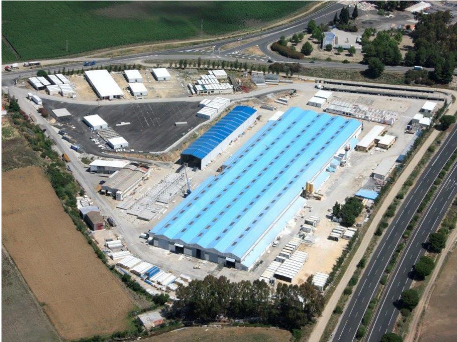
Figure 54: Industrial buildings for manufacturing and storage
