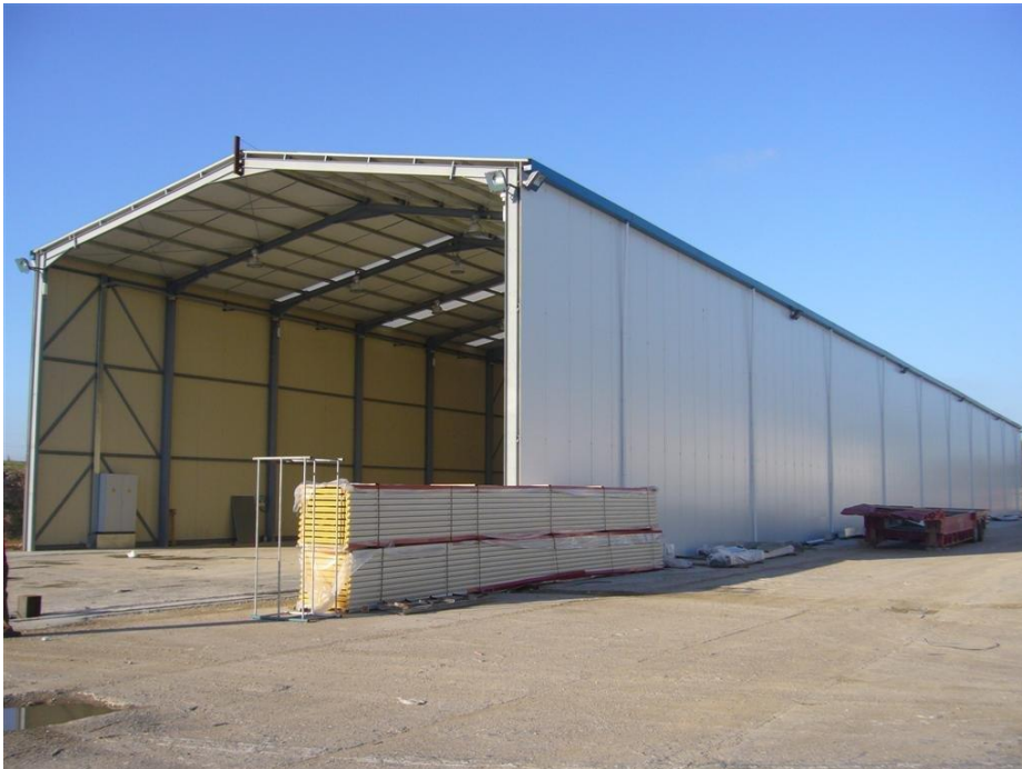
Figure 55: Industrial buildings for manufacturing and storage
