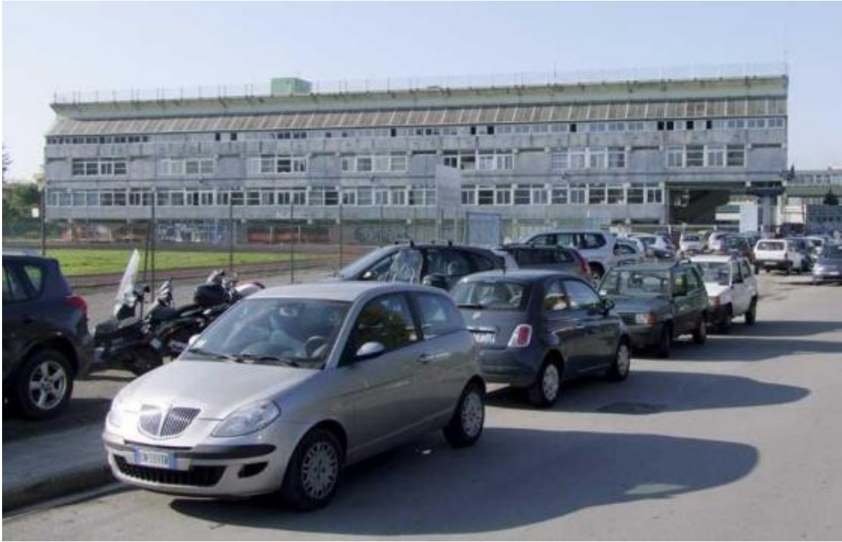
Figure 27: View of the east side
