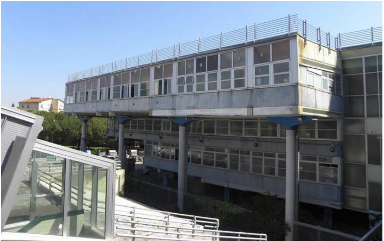
Figure 28: Partial rear view of the east side
