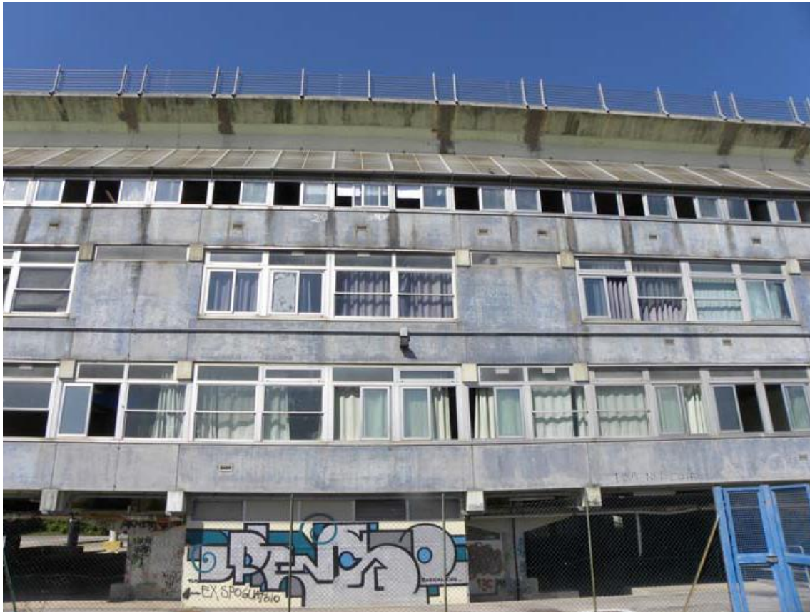
Figure 29: Detail of east side
