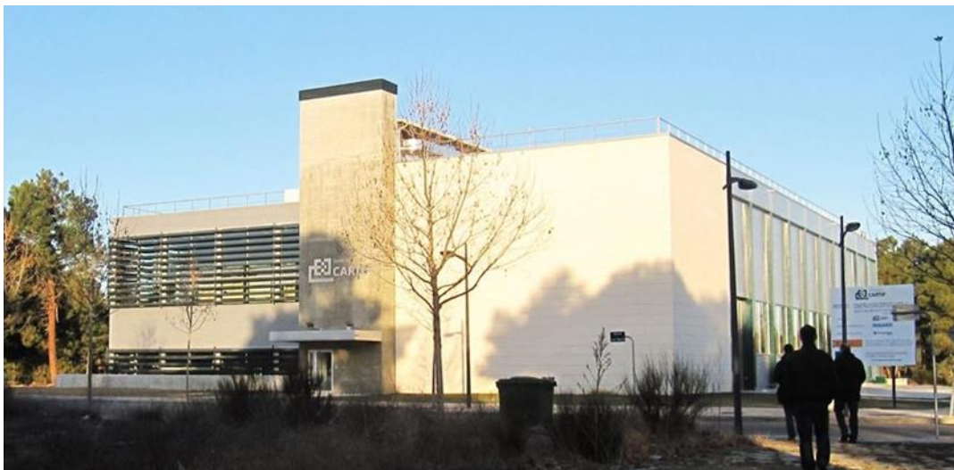
Figure 13: CARTIF-3 building; made of prefabricated modules, real scale prototypes testing facilities (chemical and industrial processes) nZEB
