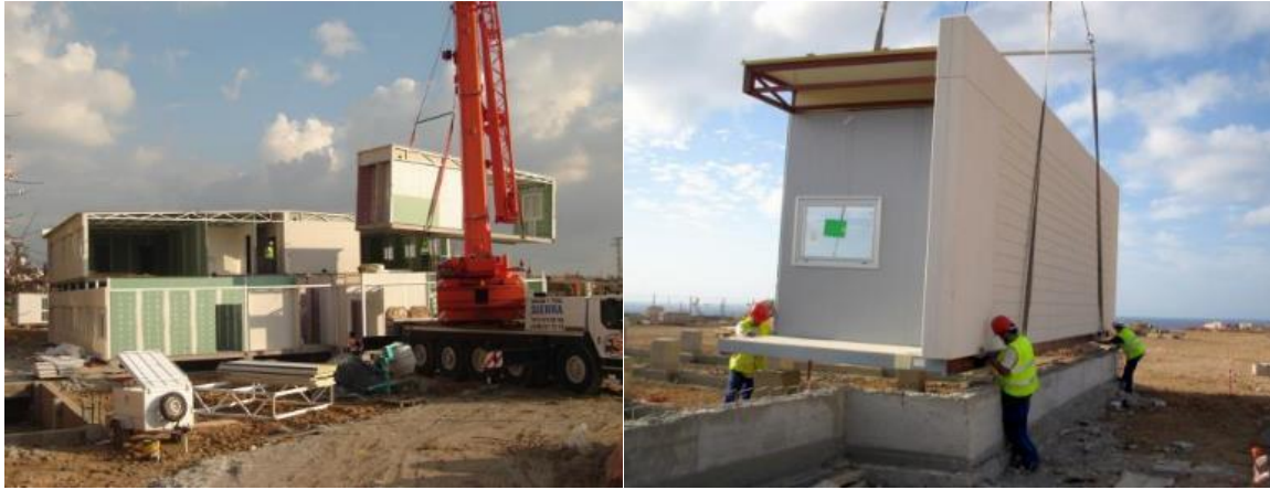
Figure 66: Modules final assembly on-site
