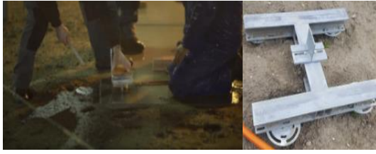
Figure 16: Reference photos from the Sustainer Homes of the tie-down locations and the reference selected foundation system
