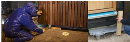
Figure 18: Reference photo from the final position between the foundation-ground floor
