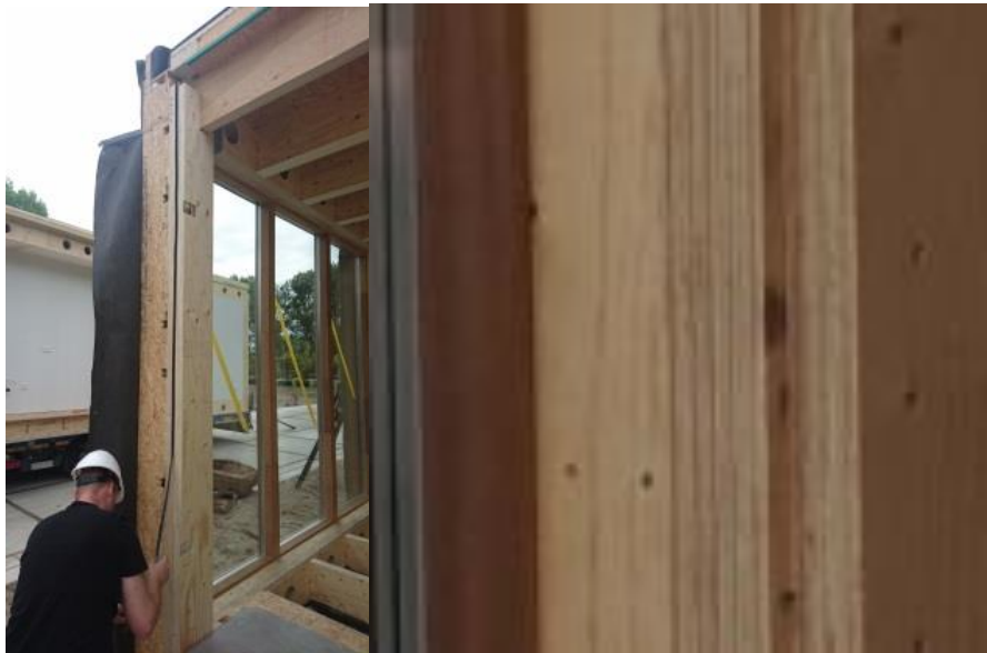
Figure 57b: Proof of the use of airtight sealant and the situation before finishing (not on the exact position of the air leak)
