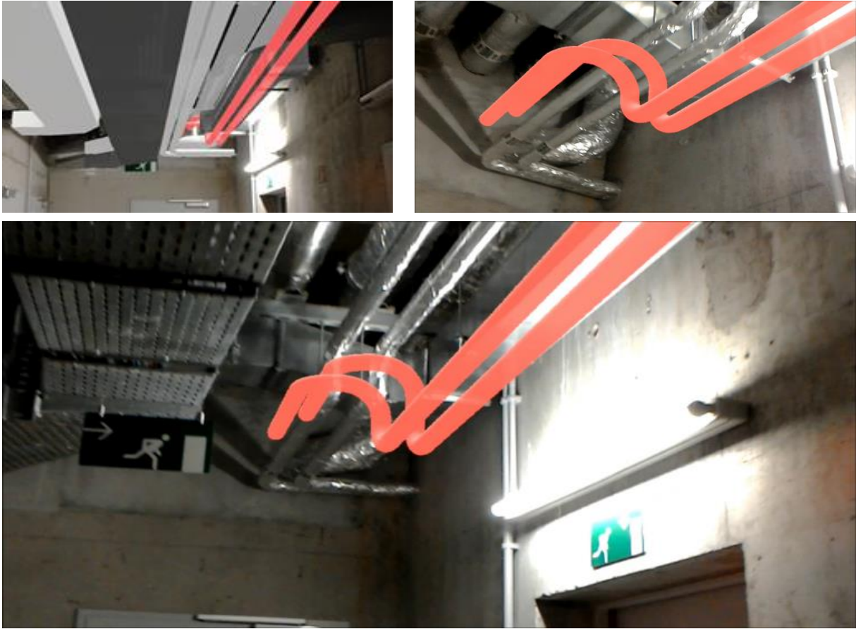
Figure 84: Visual comparison example between BIM-based MEP model and the planned-to-be target state and installation of the MEP system to be conducted at Fraunhofer example building with MS HoloLens.
