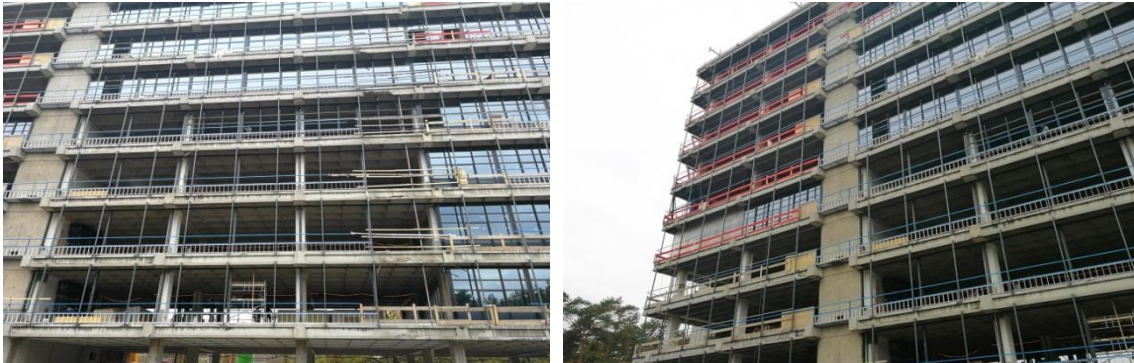
Figure 68: Current situation on-site from 14th November 2017: 1/ south corner – hotel part; 2/ south-east façade; 3/ north corner
