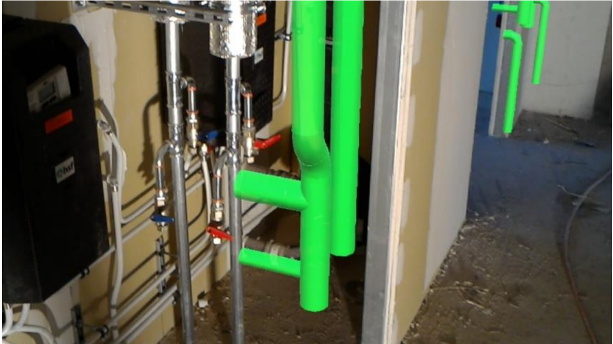
Figure 106: INSITER HoloLens BIM-based Mixed Reality App – On-Site Demonstration focus on MEP with particular visualization of one component (here: waste water system, for example)
