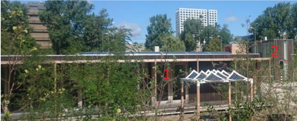
Figure 36: Office Building (1) and Student Housing (2) situation August 2018
