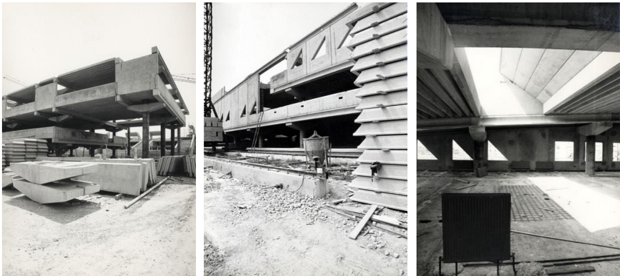
Figure 124: Pictures of the construction site of the School Complex in 1970s, showing the huge use of prefab components both for the structures and the building envelope. Below, the School Complex after completion.
