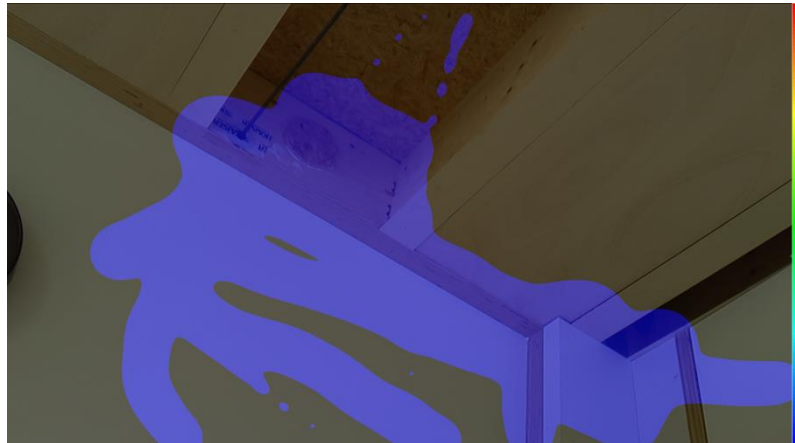
Figure 53: Ultragraphic image of the airtightness of the connection between the modules. The image shows no ultrasound attenuation through the joints of the module.
