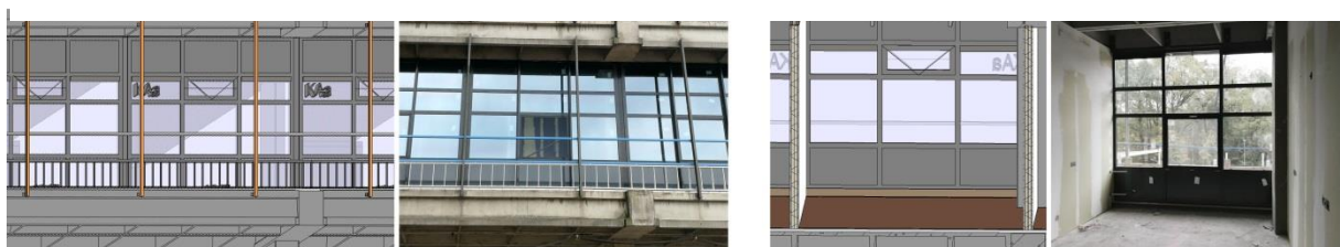
Figure 76: Comparisons between real live situation and the BIM model: general outside and inside views on the façade panels
