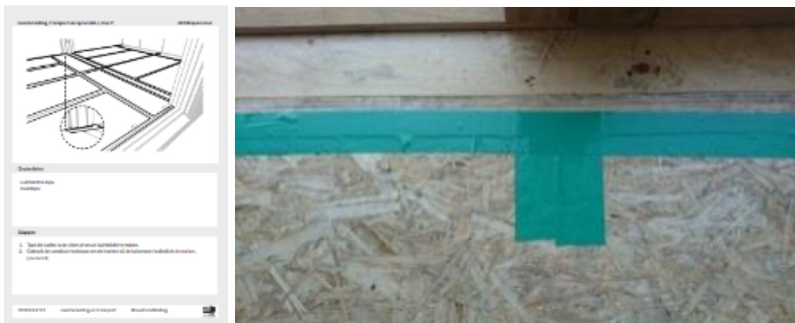
Figure 41: Adhesive tape instruction and application
