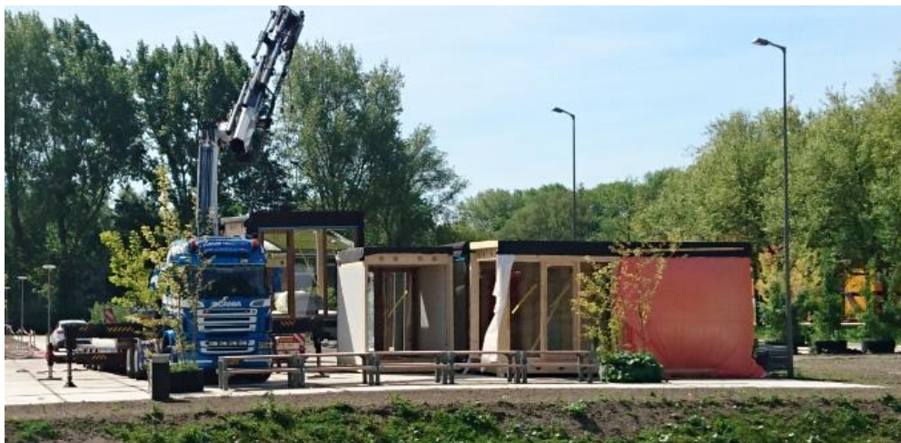
Figure 38: Delivery and storage of the modules
