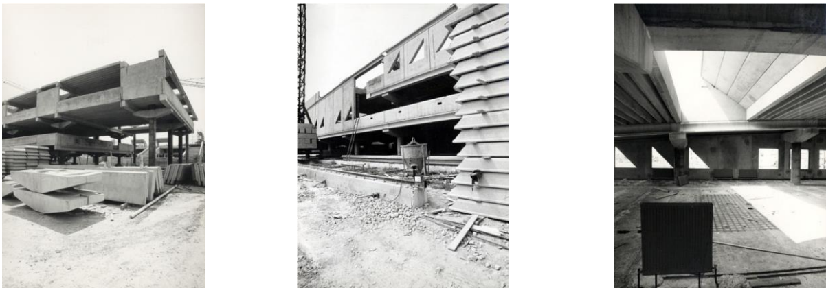
Figure 29: construction site of school complex in 1970s showing huge use of prefab components for structures and building envelope
