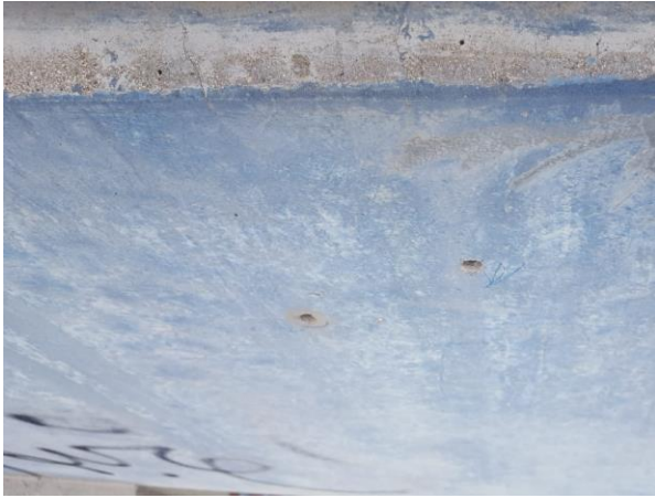
Figure 133: Drilling of the panel
