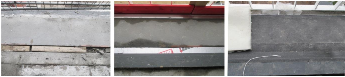
Figure 74: Work progress on the window sill at connection with the bitumen finishing
