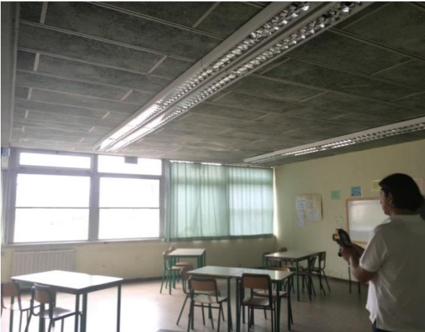
Internal view: window, opaque panel, concrete structure
