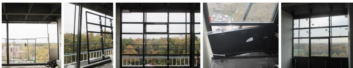
Figure 73: Work progress on installation of the façade panels: 1/ placing wooden frames; 2/ placing aluminium frames; 3/ aluminium frames; 4/ placing panels; 5/ final result
