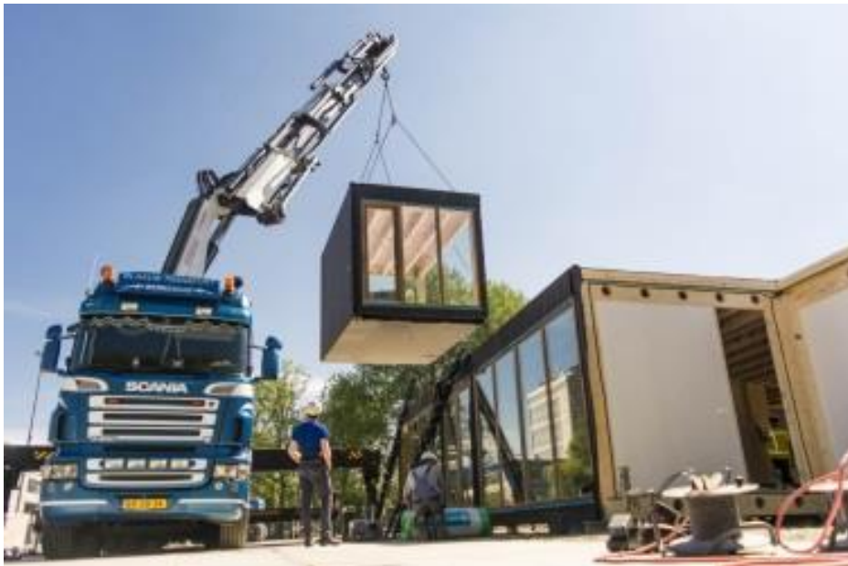
Figure 37: Placing modular elements
