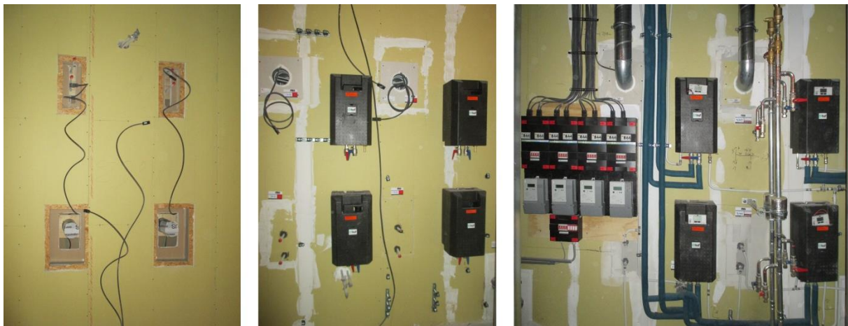
Figure 71: Work progress on the installation of the bathroom units: the meter cabinet on different stages of completion
