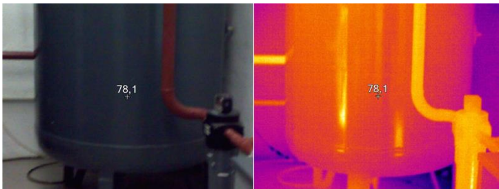
Figure 154: Thermography of the solar storage tanks
