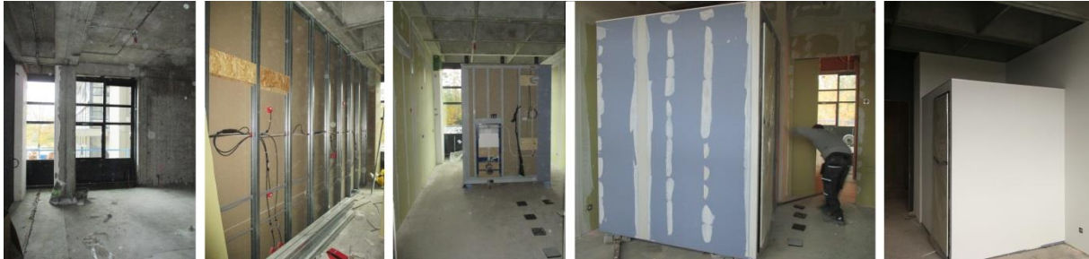
Figure 70: Renovation of a student apartment; placing of a bathroom unit: 1/ state before renovation; 2/ placing walls; 3/ placing a bathroom unit; 4/ installation of the bathroom unit; 5/ painting – state after finishing renovation
