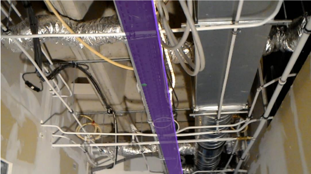
Figure 104: INSITER HoloLens BIM-based Mixed Reality App – On-Site Demonstration focus on MEP with particular visualization of one component for self-instruction or self-inspection (here: cable duct, for example)
